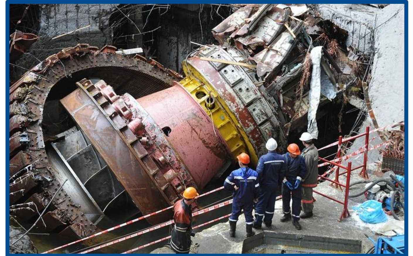
The first days after the Sayano-Shushenskaya HPP accident Photo TASS
