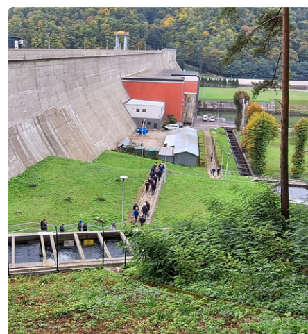
Fig. 5. The study visit participants step down along the Rożnów HP fish ladder and the dam towards the powerhouse. The view from the road leading to the Rożnów Dam
